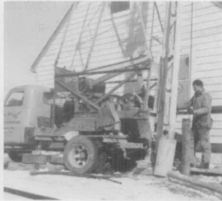
Gus Beyer of Merton, Wisconsin, drilling 6-inch suburban well near Merton.
